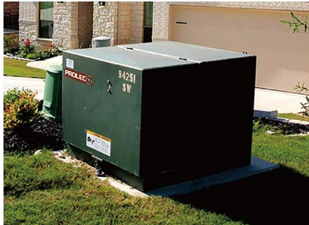
7.2kV/167kva Single phase pad mounted transformer exported
